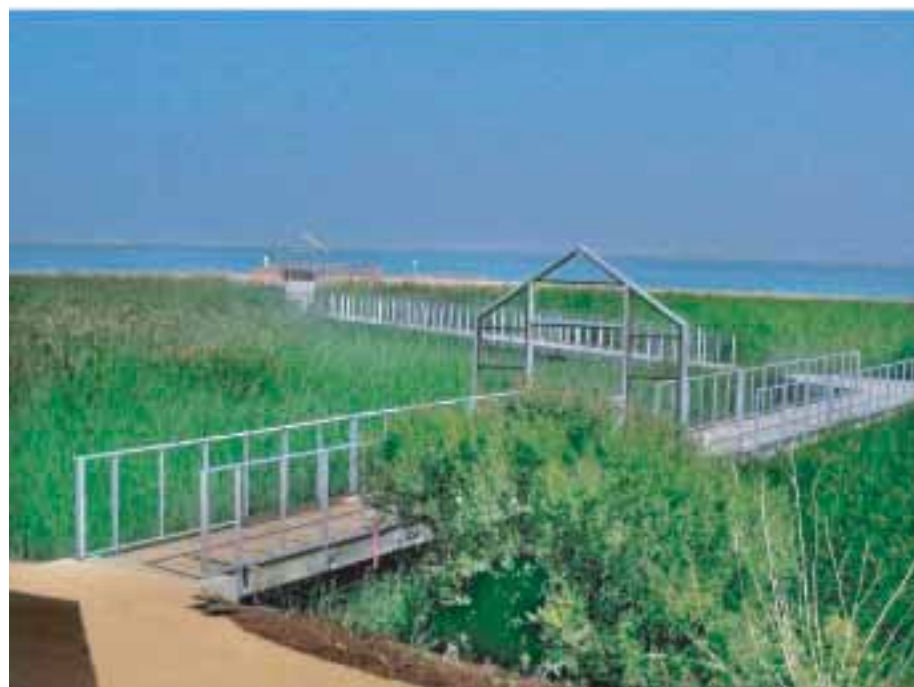
The new boardwalk spanning the Marina
